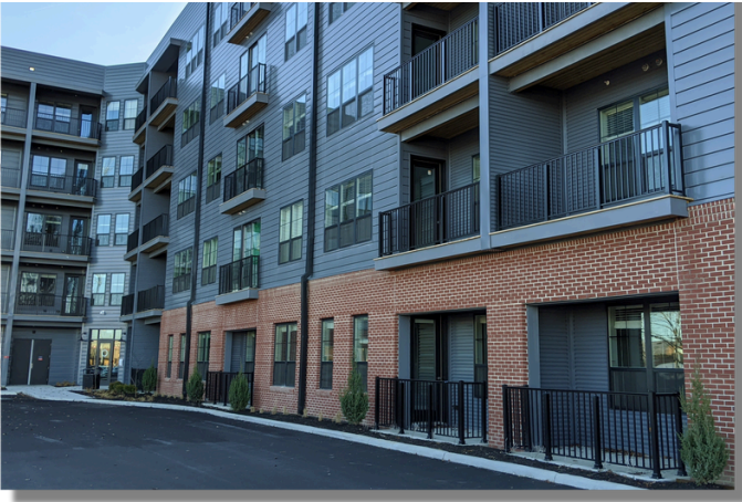
Multi-family balcony railing
